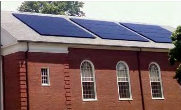
In July 2016, a photovoltaic solar system using SunPower panels was installed on the roof by BlueSel Solar, a locally owned company with offices in Woburn and Sandwich. The system will have an estimated annual output of 31,952 kWh and is expected to cover 98% of the church's electrical needs.
